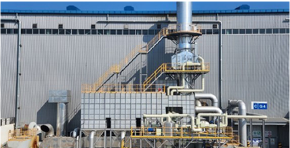
3CCL Exhaust Heat Recovery System (SeAH Coated Metal)
