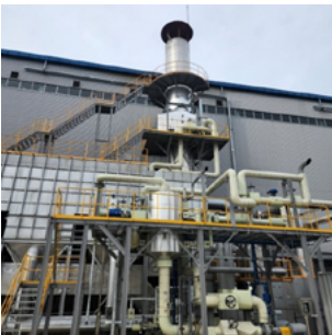
3CCL Exhaust Heat Recovery System (SeAH Coated Metal)
