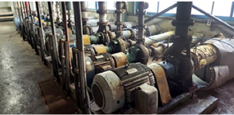
Installation of Inverter for Water Cooling Pump (SeAH Coated Metal)
